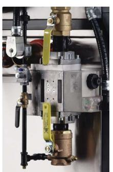
Advanced gas train design monitors and regulates gas input based on combustion air, which in turn provides highly repeatable air/fuel ratio throughout the operating range.
